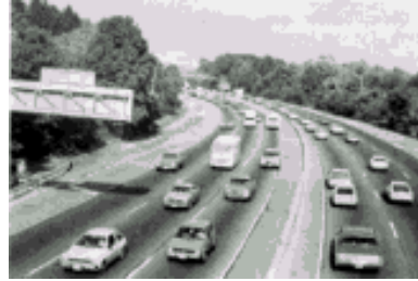
LOS D Speeds begin to decline slightly with increasing traffic levels; freedom to maneuver is more noticeably limited.
