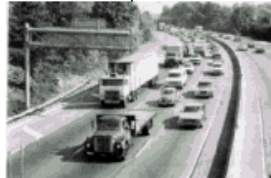
LOS E The road is at capacity; there is very little room to maneuver.
