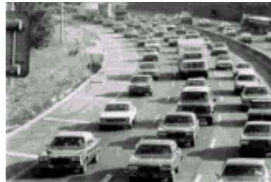
LOS F Breakdown in traffic flow; virtual gridlock.
